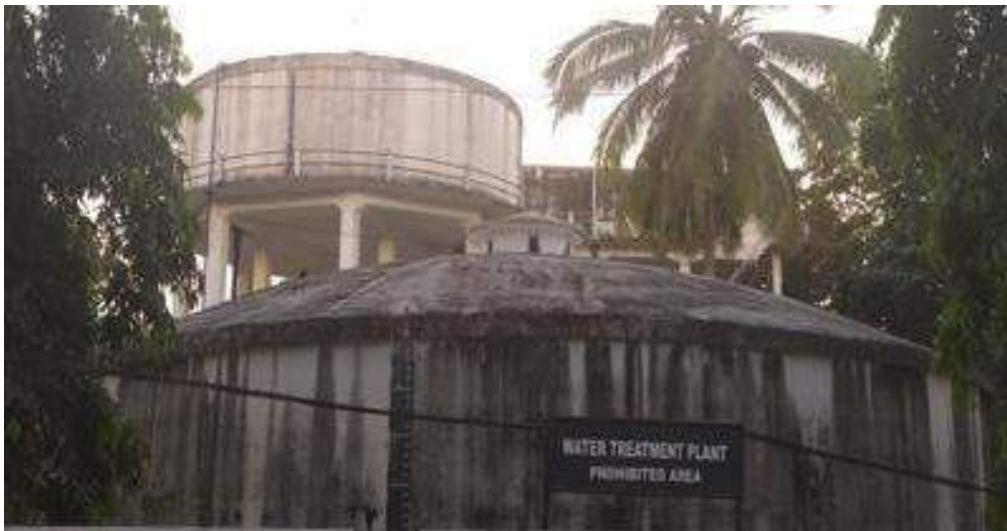
Plate 3. Water treatment facility at Calicut University Campus
