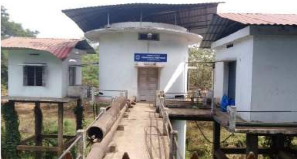
Plate 2. Pump house at Parakkadavu
